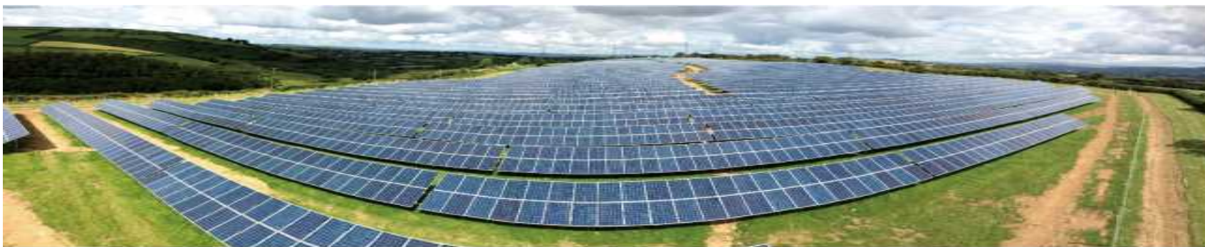
英国40MWRaventhorpe Farm地面光伏电站项目 40MWRaventhorpe Farm Ground PV Power Station, England
