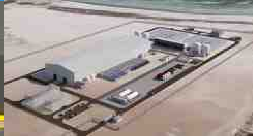
Rabigh3 132MIGD Seawater Desalination Project, Saudi Arabia
